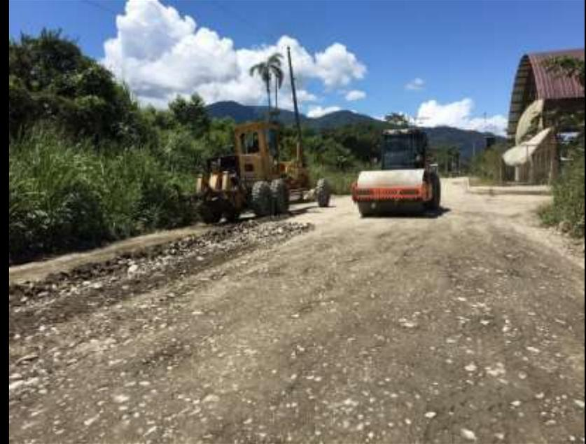
VIA SEVILLA PROVEEDURIA (TERMINACION DE COLOCACION SUBBASE Y BASE GRANULAR PREVIO AL ASFALTADO DE LA VIA ( AREA 16.300 M2) INCLUYE EL COSTO DE LA SUBBASE Y BASE.
